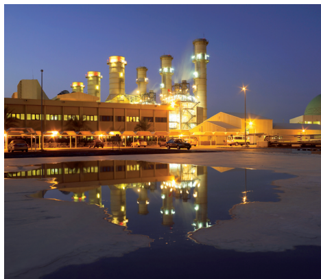
On the cover Al Taweelah 1068-MW combined cycle desalination plant in Abu Dhabi, powered by three Siemens SGT5-4000F gas turbines
